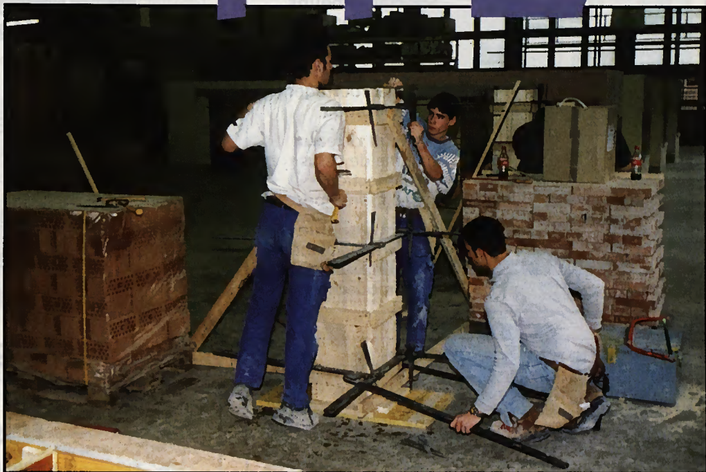
Halle de construction. PHOTO FFE
