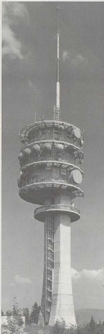
Weather visible: the telecommunication tower on Gibloux
